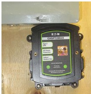
A surge protection device mounted on a residential circuit breaker panel
