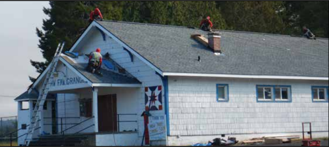
After 4 years of fundraising, we at Baw Faw Grange were finally able to get our new roof, fascia and gutters put on!!
